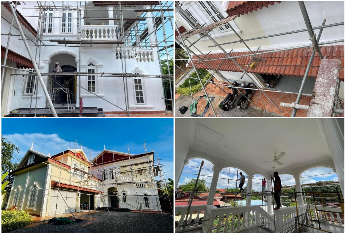
Renovating the JGG dormitory in Siem Reap
