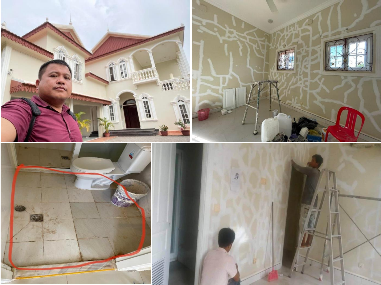
Renovating the JGG dormitory in Siem Reap
