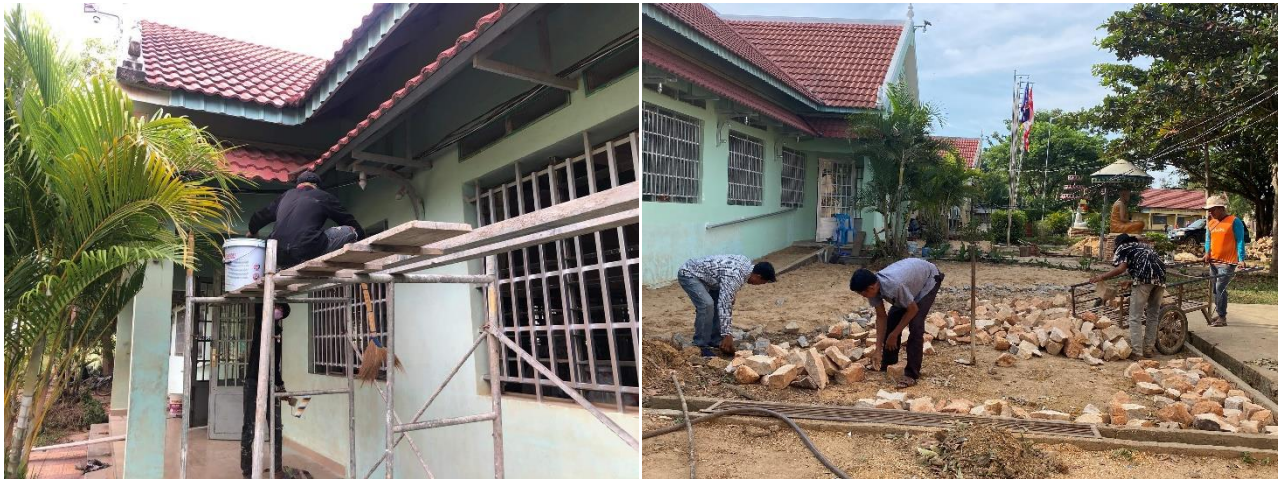
Repairing, Repainting and Cement concreting Bakchinhchien Hun Sen High School
